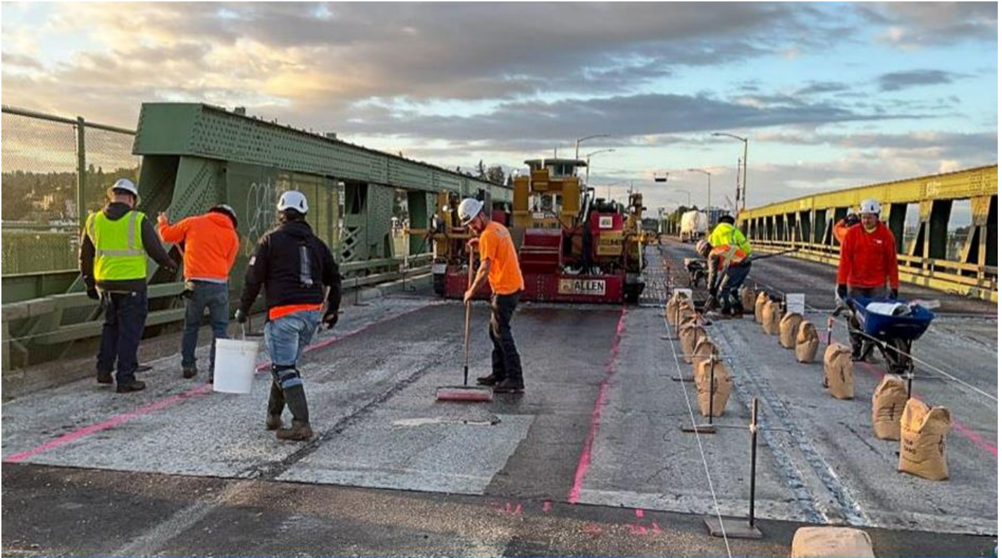
Program 9 – On the Ballard Bridge, crews prepare to apply polyester polymer concrete as part of the 15 th Ave NW/Ballard Bridge Paving and Safety Project.
