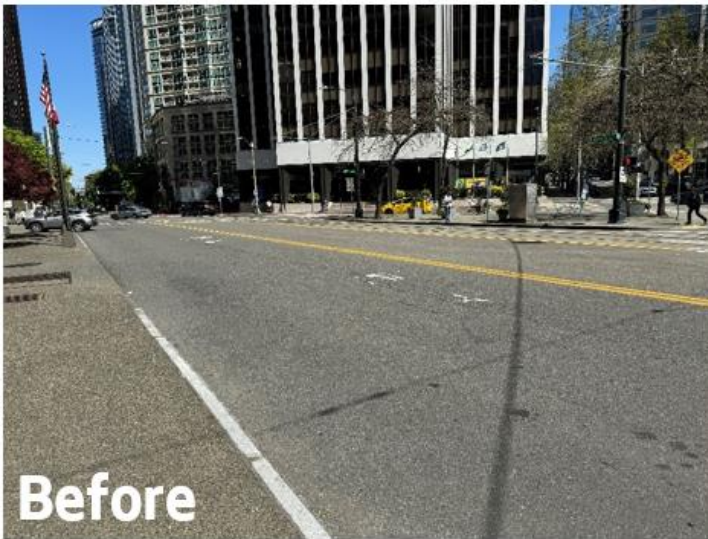
Program 21 – Before and after a transit spot improvement on Westlake Ave and Stewart St. Before this improvement, cars coming out of the Westin Hotel were making left turns onto Westlake Ave which led to several near collisions with the Streetcar. The new tuff posts prevent cars from making left turns onto Westlake Avenue.
